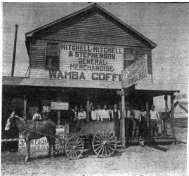
10. Stephenson's Store, the oldest building still standing in Pelly.
