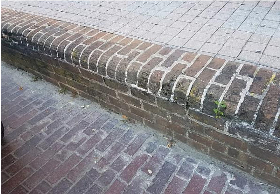
Fig 34. Cedar Bayou brick in the 24th Street curb built by Hugh Pritchard in 1874.
