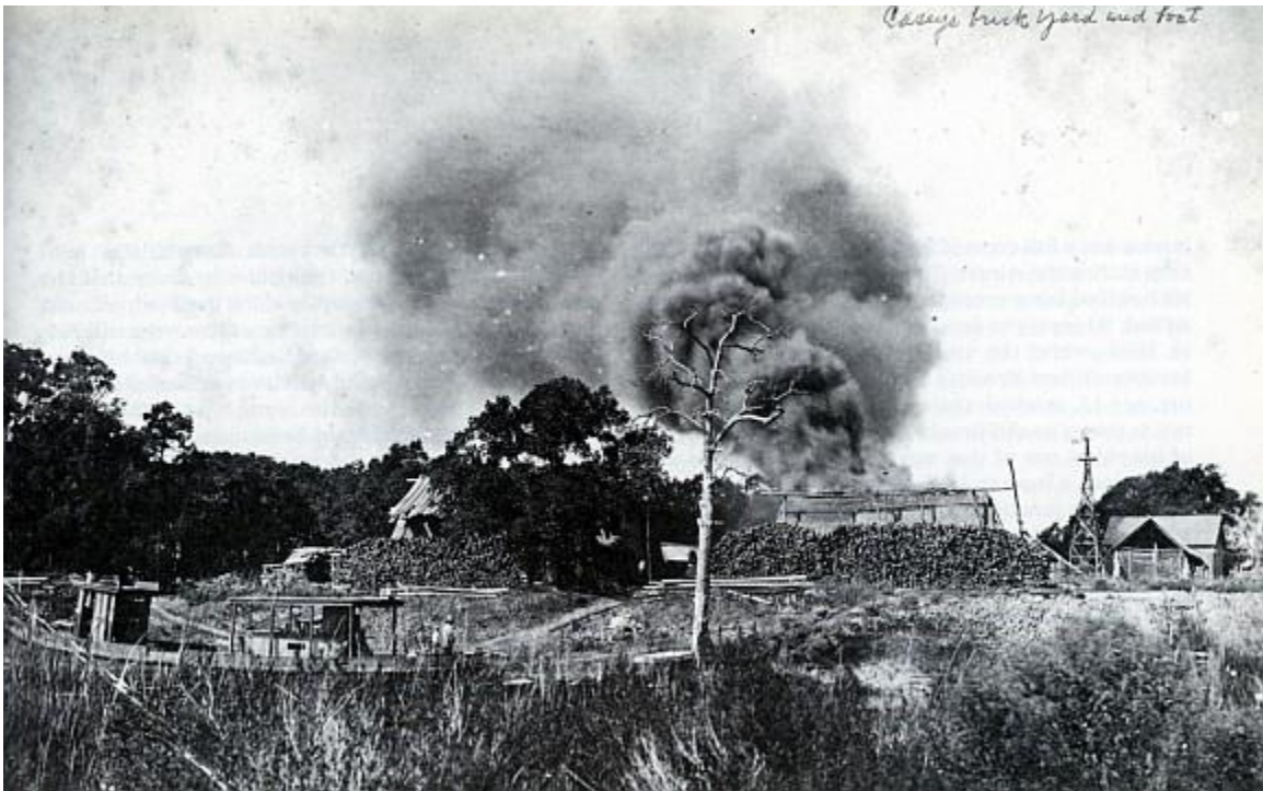
Fig 12. Mike Casey Brick Yard, 1914. The picture was taken from the Chambers County side looking across Cedar Bayou. The drying shed is just right of the windmill and a pug mill is visible between the windmill and woodpile. Sterling Municipal Public Library
