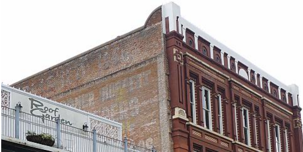
Fig 36. The 1884 W. L. Moody Building. Cedar Bayou brick on the side wall. The façade is overlaid with pressed brick. Image by author.
