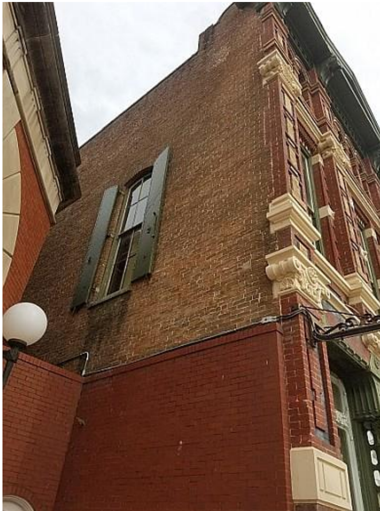
Fig 37. The H.M. Trueheart Building built by Robert Palliser at 212 22nd Street, 1882. Cedar Bayou brick is overlaid with pressed brick on the façade and first floor side wall. Image by author.
