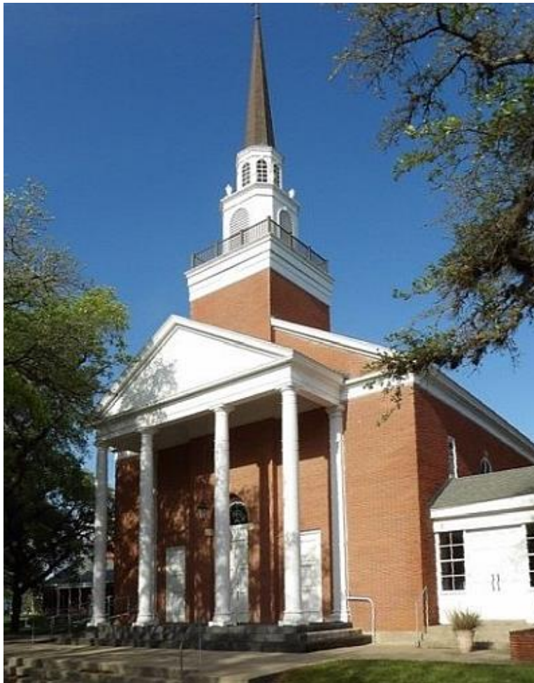
Fig 56. Cedar Bayou Methodist Church, 1953. One of the last buildings constructed with Cedar Bayou bricks. Stone-Tex Roman bricks were used on the church and on the parsonage next door. Image from internet.
