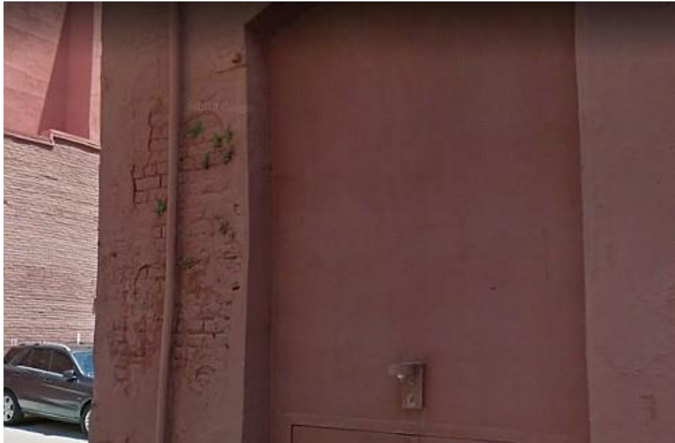
Fig 33. The Stewart Title Building, NE corner showing exposed brick.
