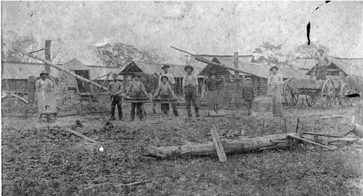
Fig 11. Wright's Brick Yard, ca 1900. Note the two pug mills, drying sheds, brick molds held by the boys, and the broken home-made pug-mill shaft in the foreground. From the collection of Kenny Wright.
