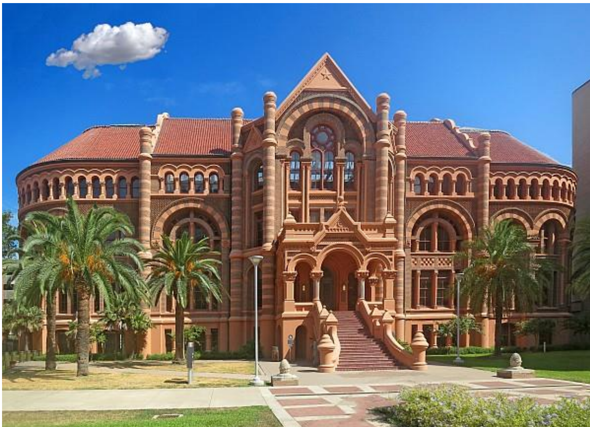
Fig 39. "Old Red", the Ashbel Smith Building at UTMB, 1891. Built by Robert Palliser and reported in the Galveston Daily News as constructed with both common and pressed brick made on Cedar Bayou. Image from internet.
